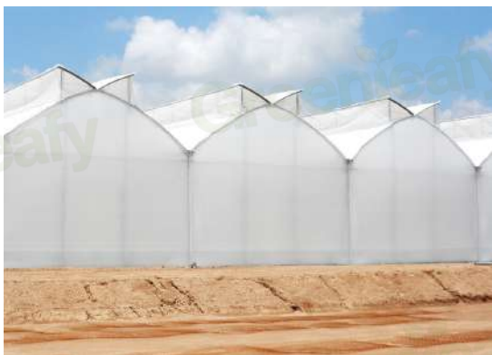
Sawtooth multi-span greenhouse
